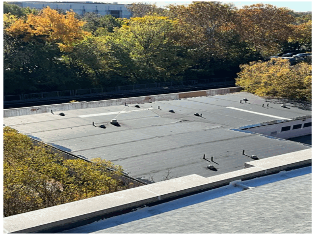
Asset X020 - Roof 1 Southeast View
