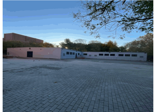
Facades A, F and E - East View
