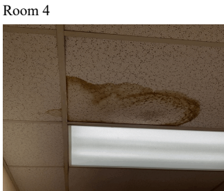
Corridor near Room 4
