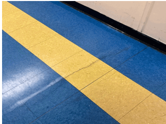
Corridor near Room 2
