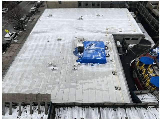
Roof 1 - South View from Asset X009
