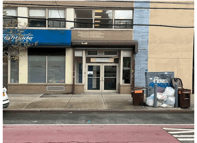
Facade A - Webster Avenue
