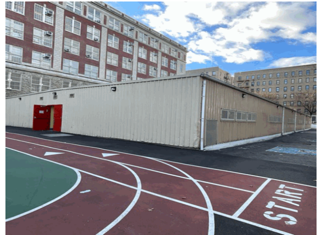
Bronx Boulevard - Northwest View
