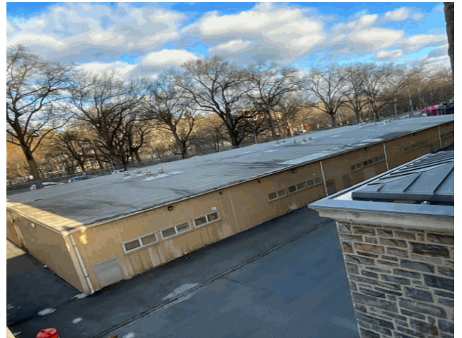
Roof 1 - Northwest View
