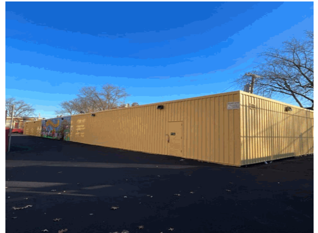
Facade A and D - Northeast view
