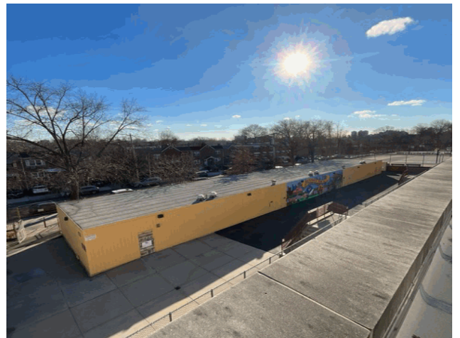
Roof 1 - South View from Main Asset X121
