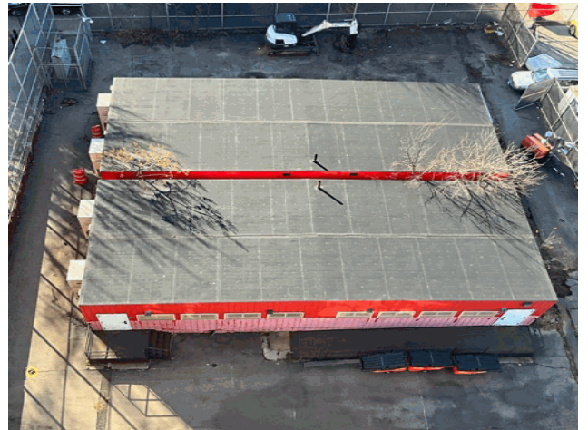
Roofs 1 and 2 from Main Asset X470
