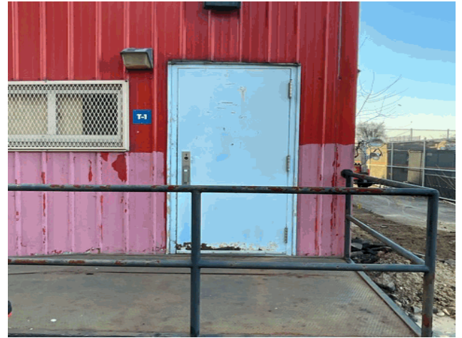
Facade A - Classroom T1
