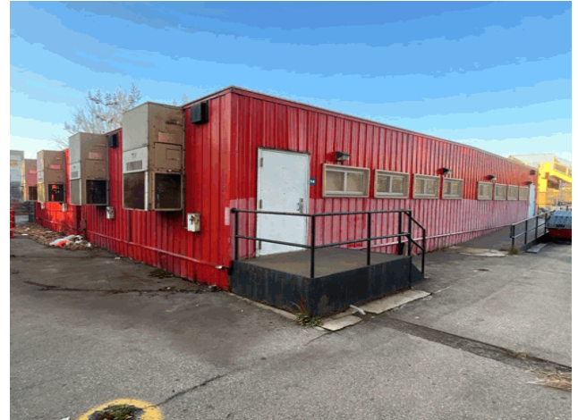
Facades B/A - Southwest View
