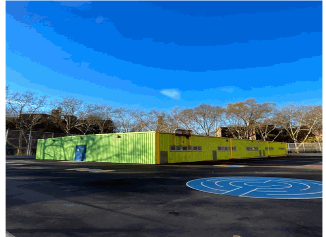
Facades A and D - Southwest View
