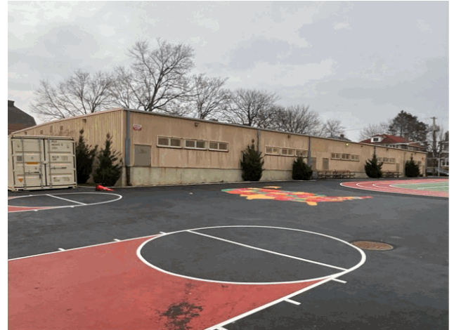
Facade B and C - Northwest View
