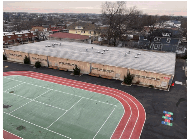
Roof 1 - Northwest View
