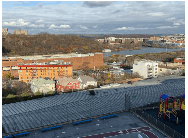
Roof 1 - Northeast View from Asset X109
