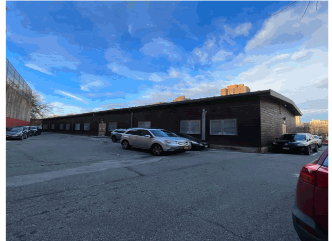
Facades A and D - Southwest View
