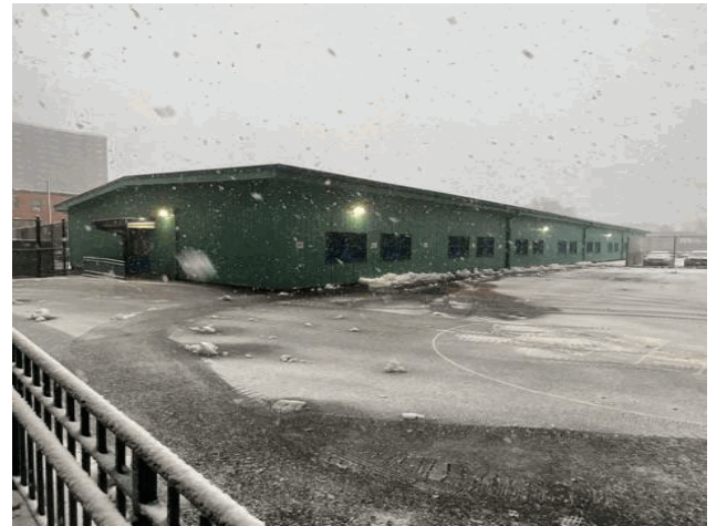
Facade A and D - Northwest View
