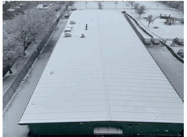
Roof 1 - North View
