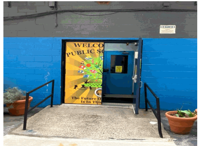
Exit 1 - Facing Main Asset
