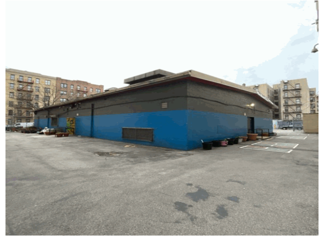
Facade A and D - Northeast View
