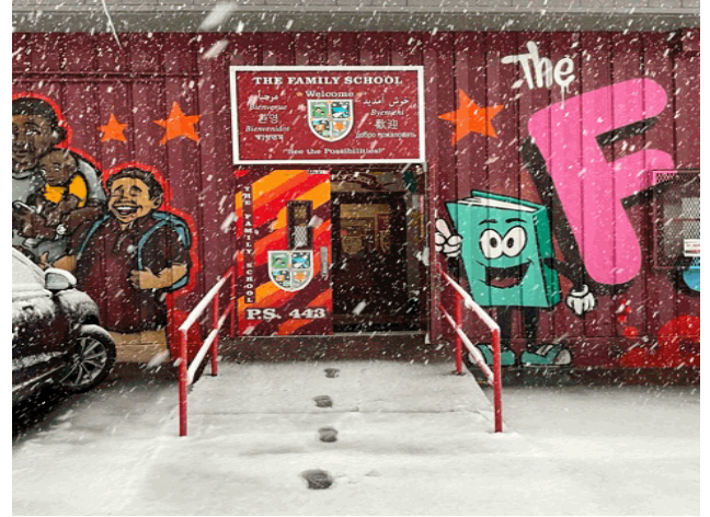
Facade A - View from Main Asset (X090)
