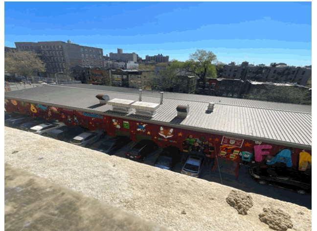
Roof 1 - East View from Main Asset X090
