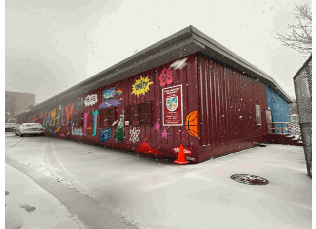
Facade A and D - Northeast View
