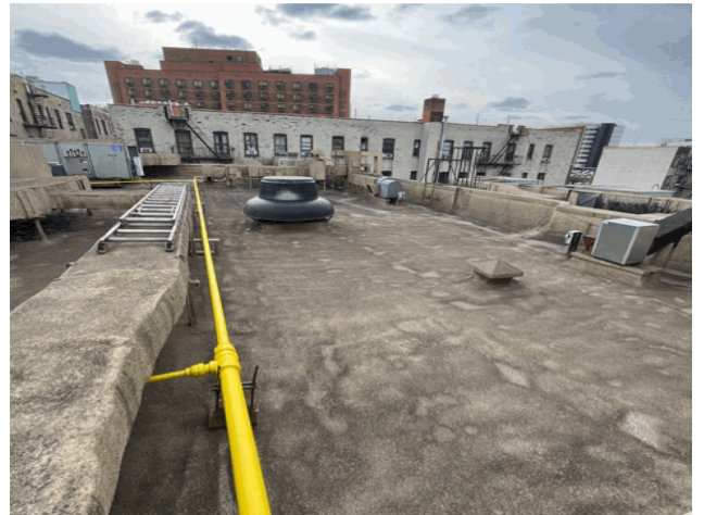
Roof 1 - South View
