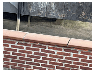
Roof 2 at Facade H
