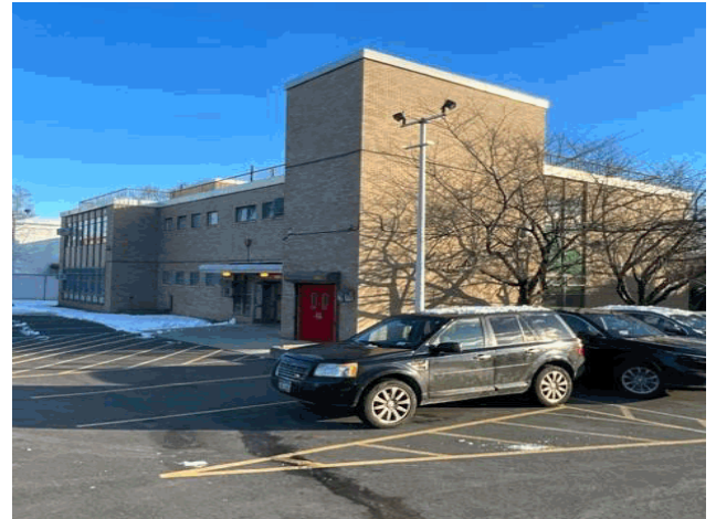
Facade A and D - North View
