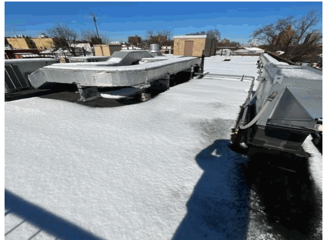
Roof 1 - North View
