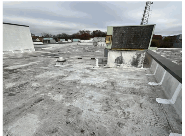
Roof 1 - North View
