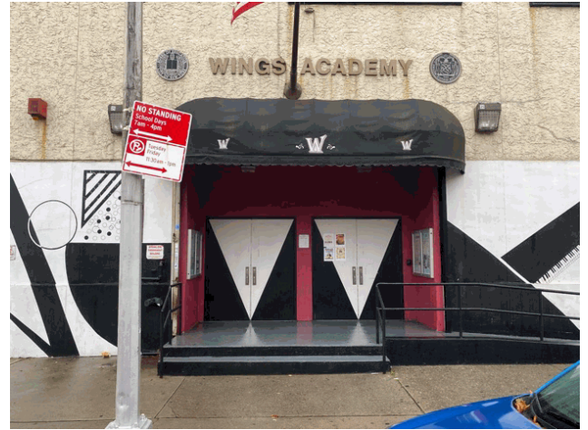
East 180th Street - Facade A
