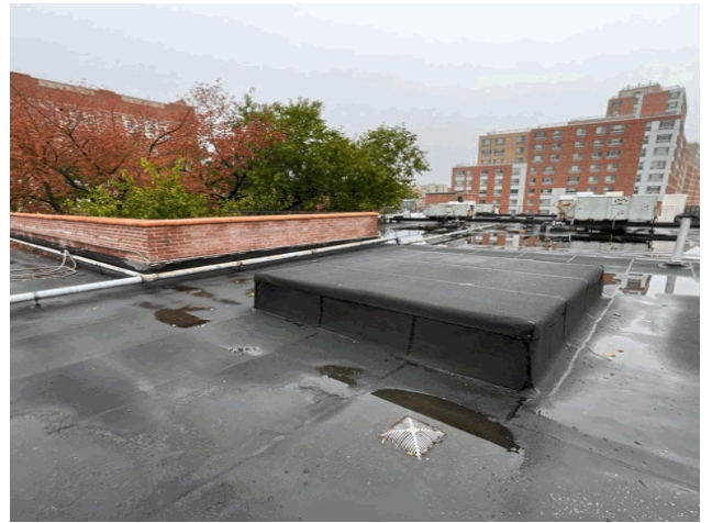
Roof 1 - North View
