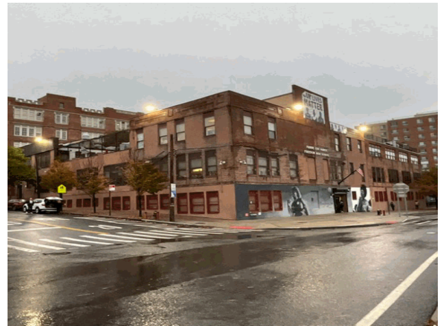
Corner of Jennings Street and West Farms Road - Southeast View
