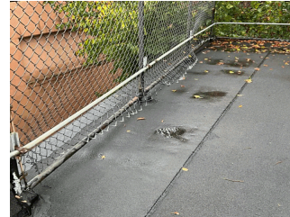
Roof 1 - Facade E
