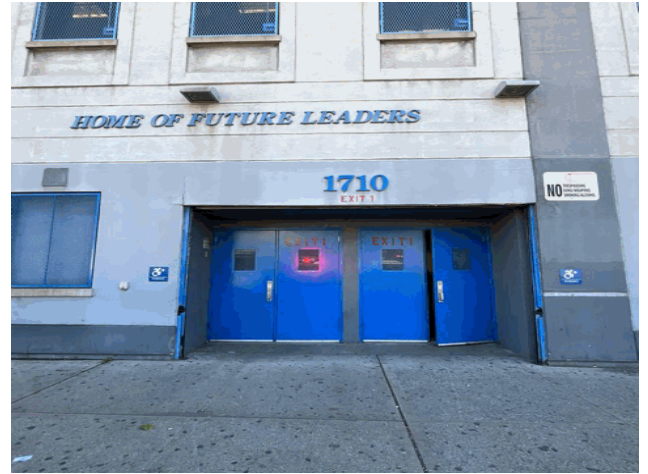
Facade A - Webster Avenue
