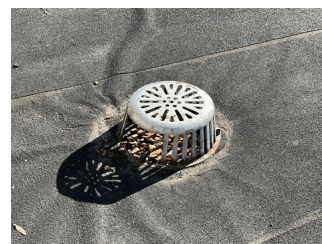
Roof 1 - Facade B
