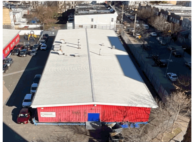
Roof 1 - North View from Main Asset X053
