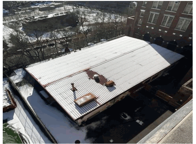
Roof 1 - South Viewed from Main Asset X073
