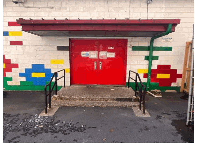
Facade A - Facing Main Asset
