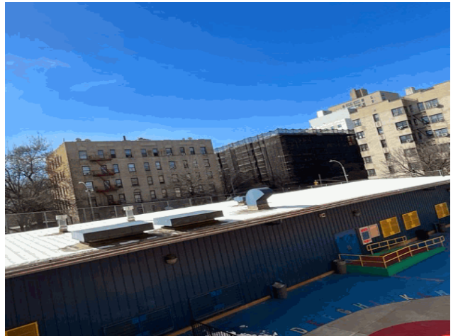
Roof 1 - South View from Main Asset X070
