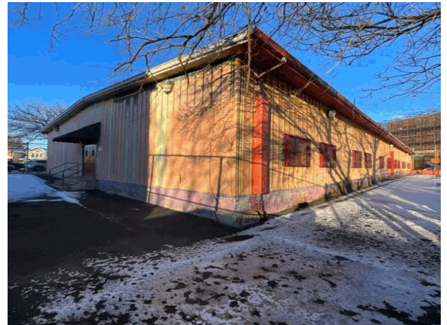
Facades B and C - Northwest view
