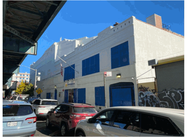
Jerome Avenue- Northeast View
