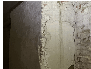
Stair from 2nd Floor to rear
