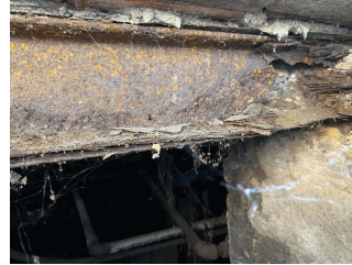
Beam above Basement access door
