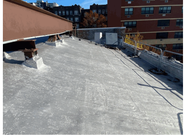
Roof 1 - East View
