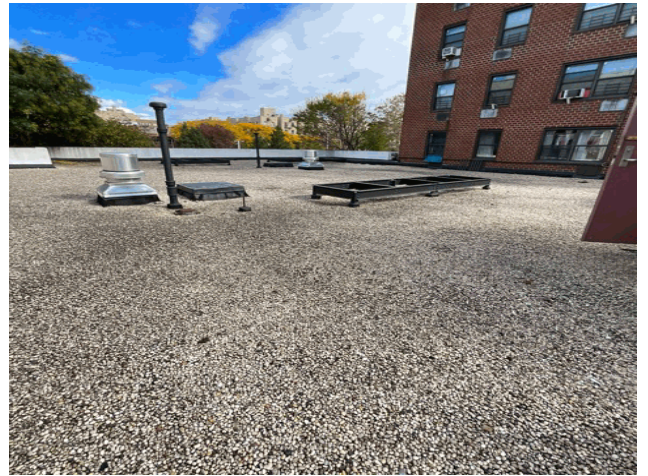
Roof 1 - East View
