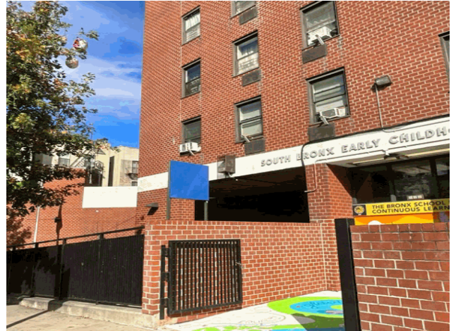
East 139th Street - Northwest View
