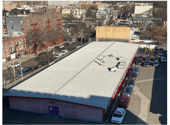
Roof 1 - North View from Main Asset X053
