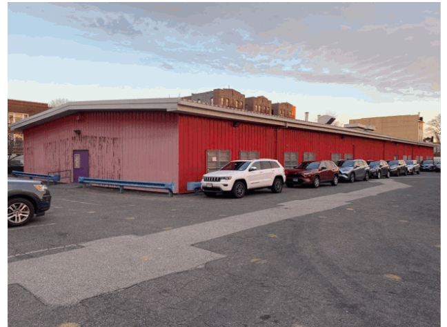
Facade A and B - Northwest View
