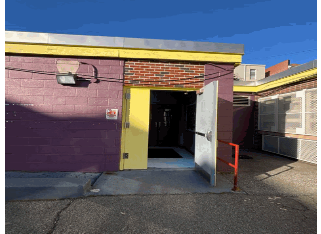
Facade A - Coster Street
