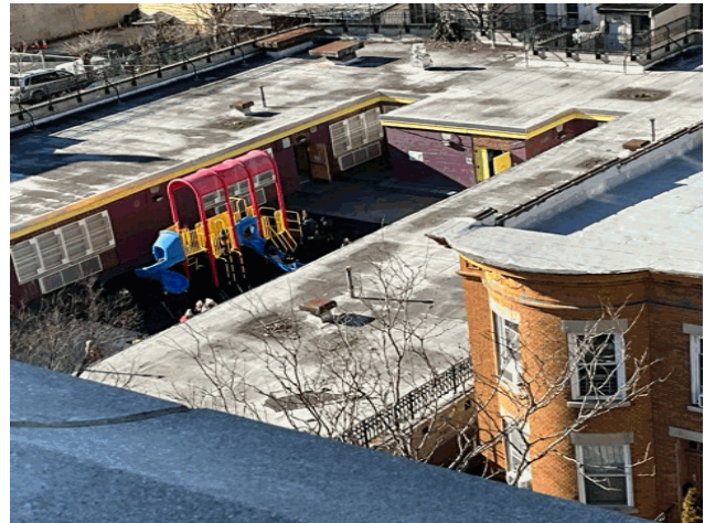
Roof 1 - Southwest View from Main Asset X048
