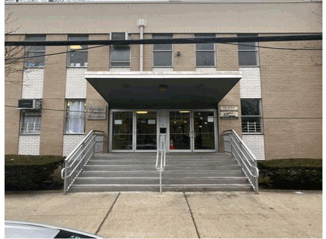
Facade A - Hillman Avenue
