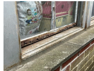
Facade B (AW1)
