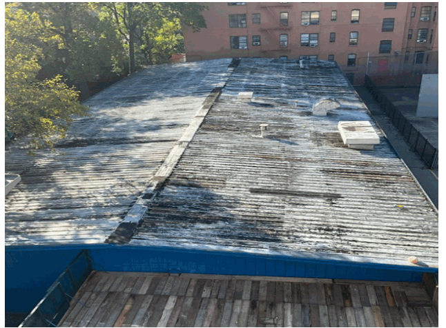
Roof 1 - South View
