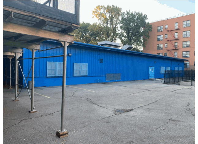
Facade A - Southeast View
