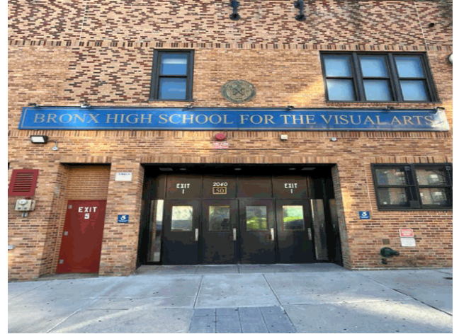
Facade A - Antin Place
