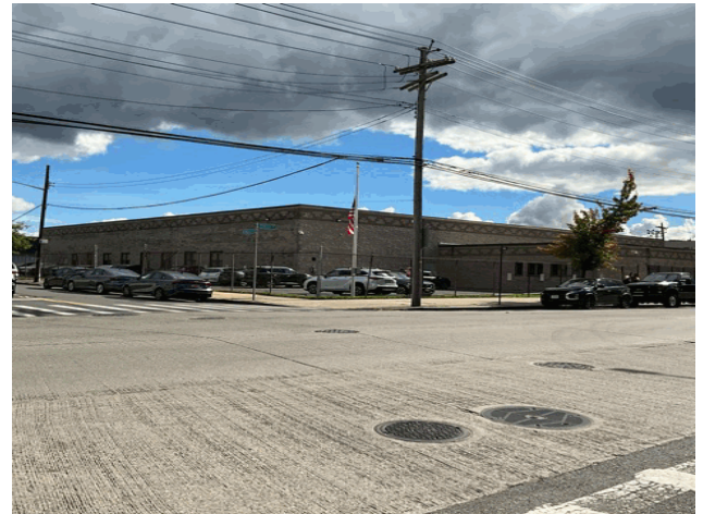
Corner of Zerega Avenue and Ellis Avenue - Northeast View
