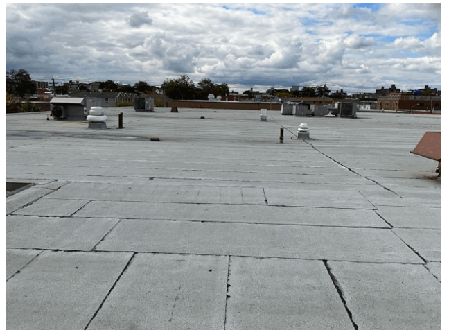
Roof 1 - Southwest View
