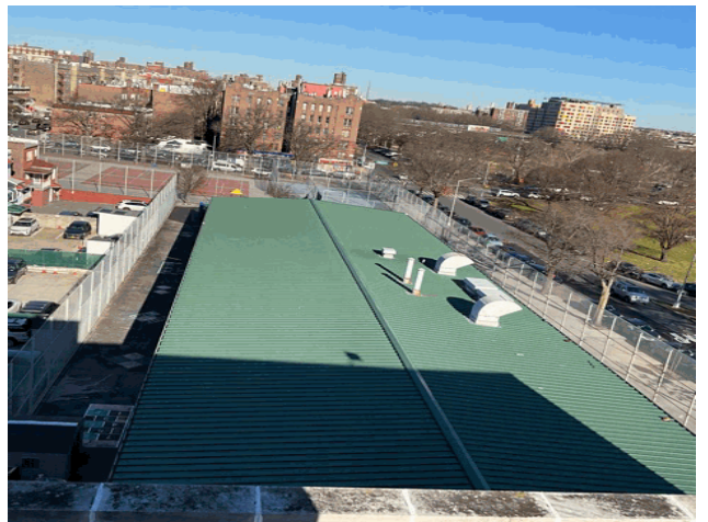
Roof 1 - North View from Main Asset X123
