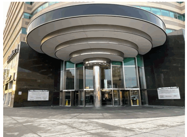
Facade A - Fordham Room
