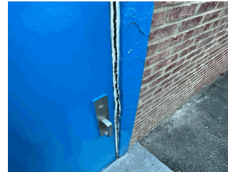
Facade F (exit door)
