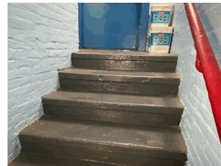
Exit 2 Vestibule and Stair to Basement
