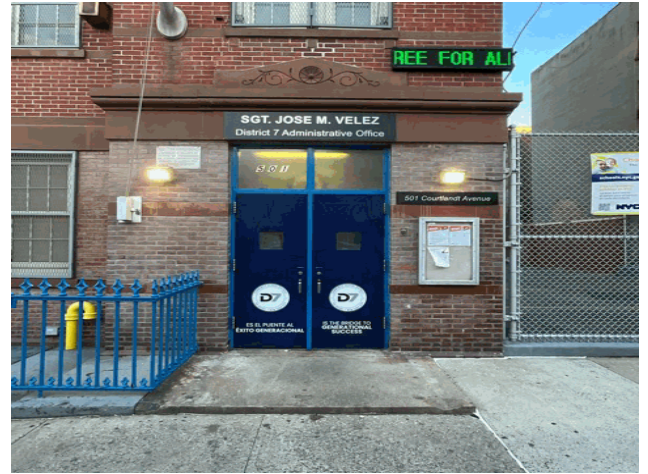
Facade A - Courtlandt Avenue
