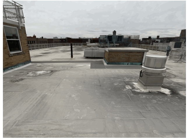
Roof 1 - South View
