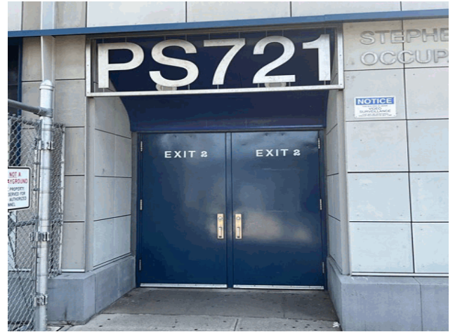
Facade A - Walter Avenue
