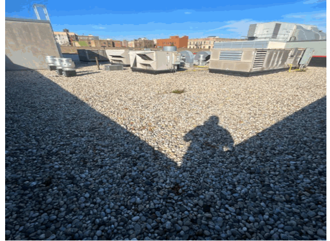
Roof 1 - Northwest View
