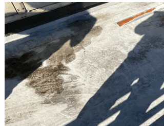
Roof 3 - Plaza Deck
