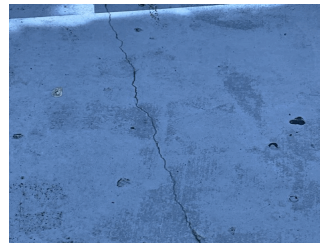
Roof 3 - Plaza Deck
