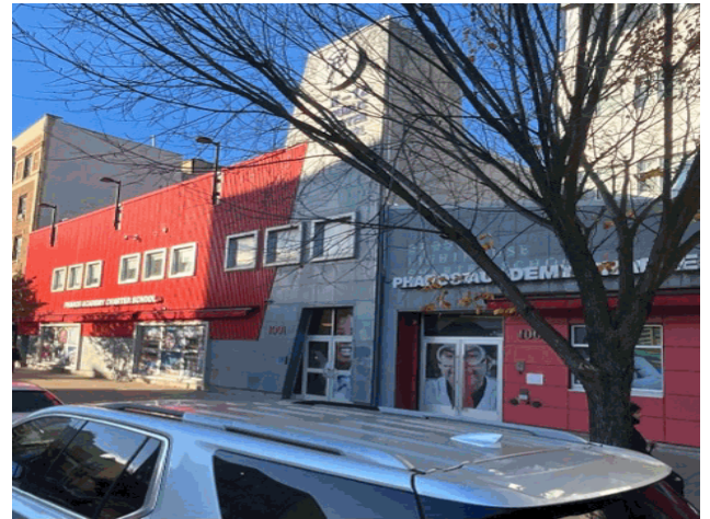
Intervale Avenue - Southwest View
