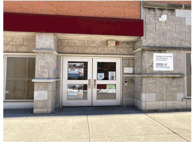
Facade A - Ogden Avenue
