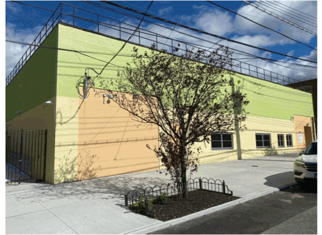
East Gun Hill Road - Northeast View
