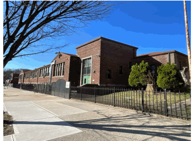
Dyre Avenue - East View
