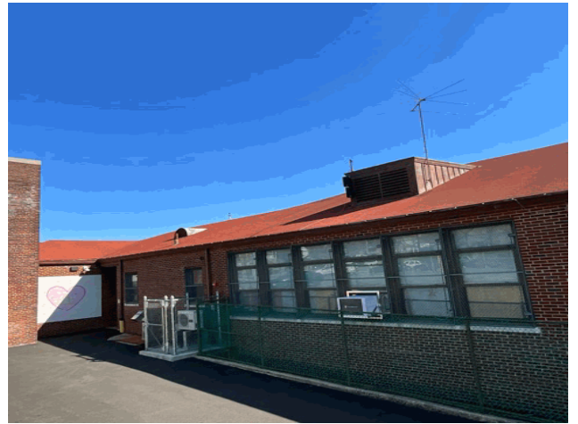
Roof 1 - West View
