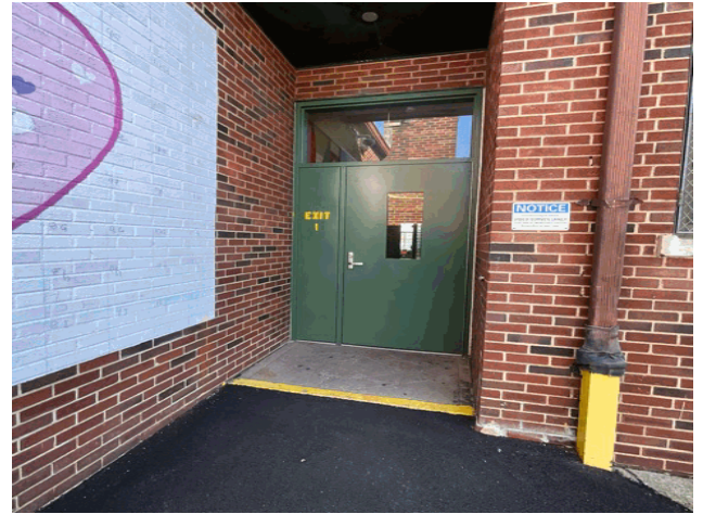
Facade F - Facing parking lot
