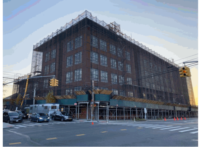
Corner of Bronxdale Avenue and Van Nest Avenue - East View
