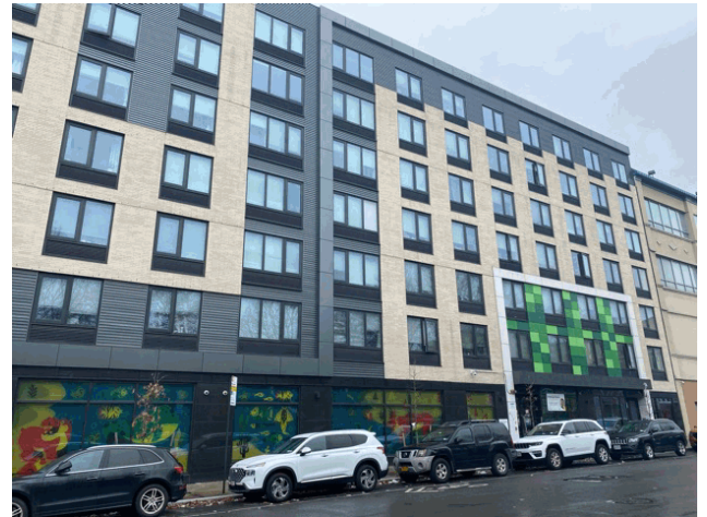
Third Avenue - Northwest View
