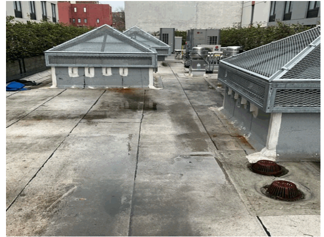
Roof 1 - North View
