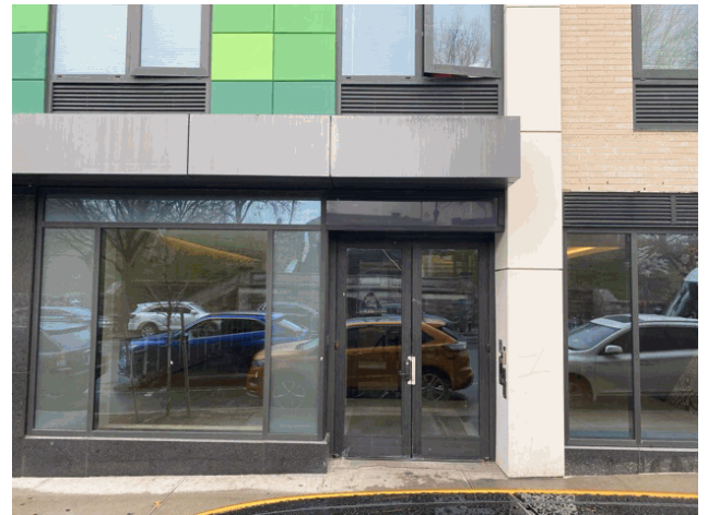
Facade A - Third Avenue
