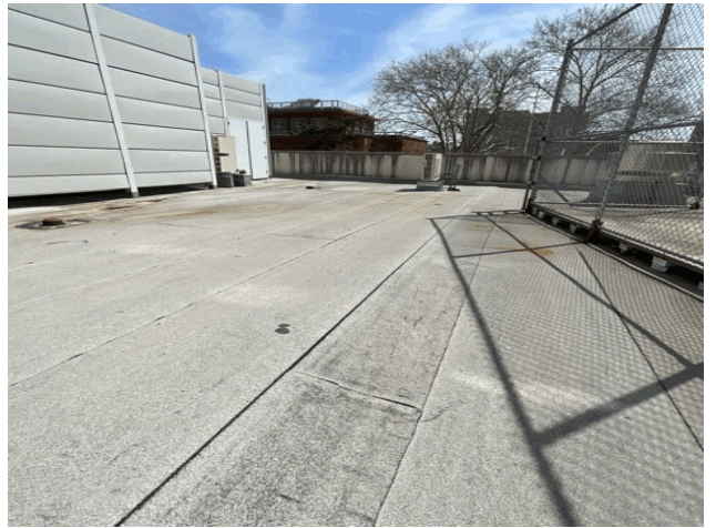
Roof 1 - North View
