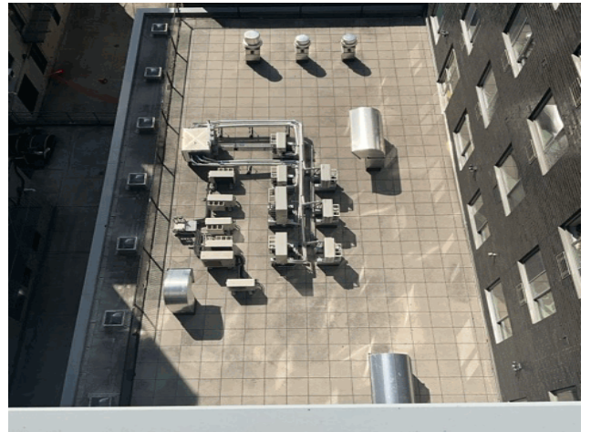
Roof 1 and Plaza Deck - South View
