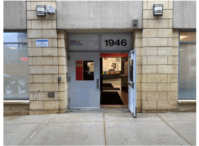
Facade A - Boston Road
