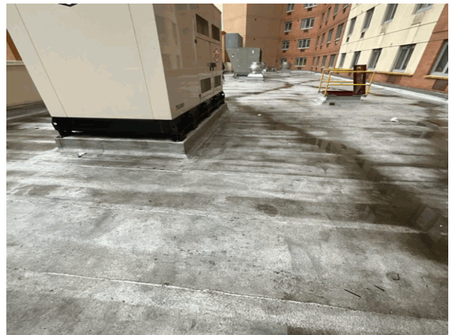
Roof 2 - North View
