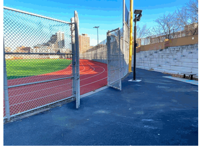
Facade A - Northeast View
