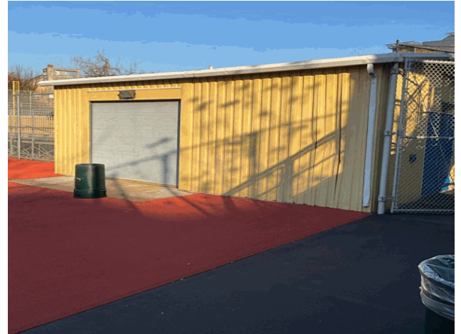
Facade F - Northwest View
