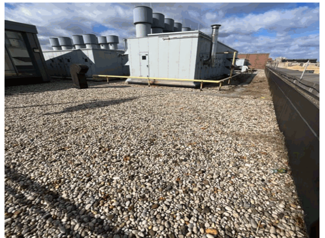
Roof 1 - West view
