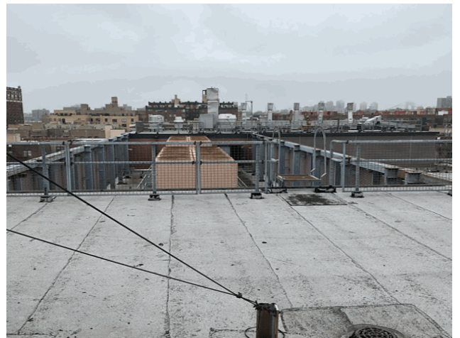
Roof 2 - Northwest View
