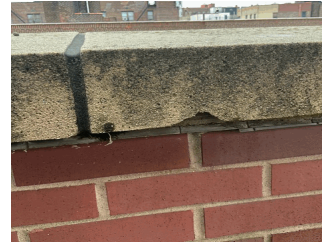
Plaza Deck 1 at Facade D
