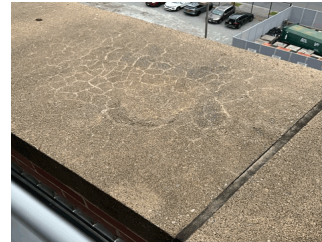
Plaza Deck 1 at Facade C
