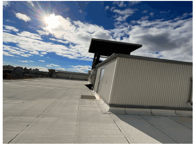
Roof 1 - Southwest View
