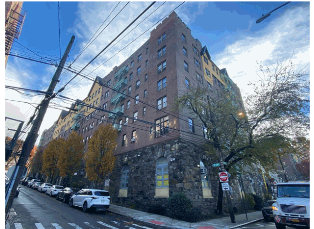
Corner of West 228th Street and Cannon Place - South View
