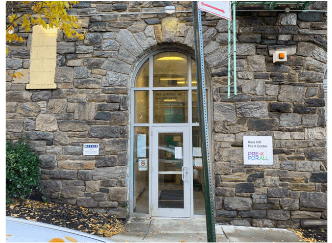
West 238th Street - Facade A
