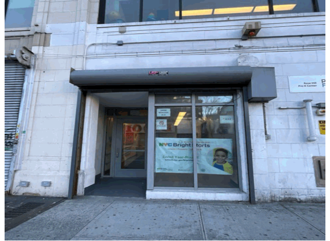
Facade A - Webster Avenue
