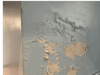
Stair E/1 Near Exit 13
