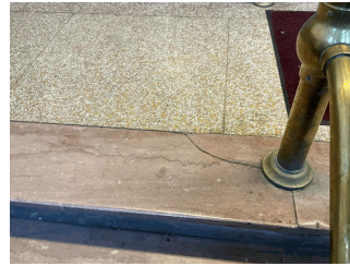
Main Entrance Lobby
