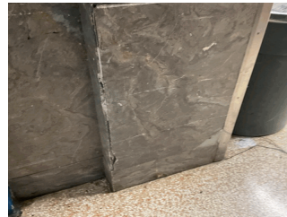
Main Entrance Lobby
