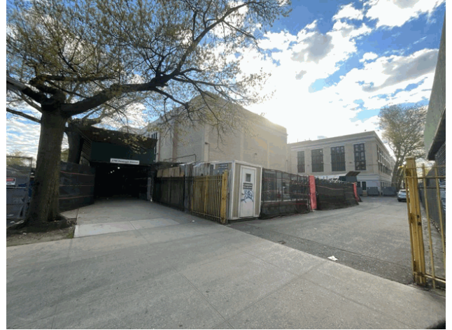
Corner of Reservoir Ave and Lehman Walking Roads - North View
