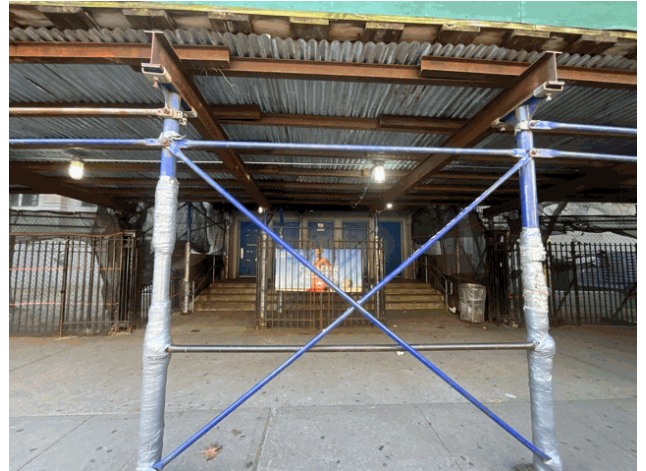
Facade N - Reservoir Avenue
